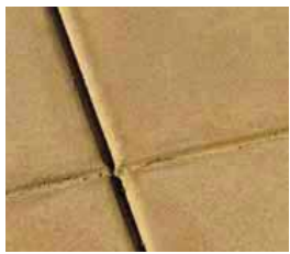
Groove Tooled Joints
